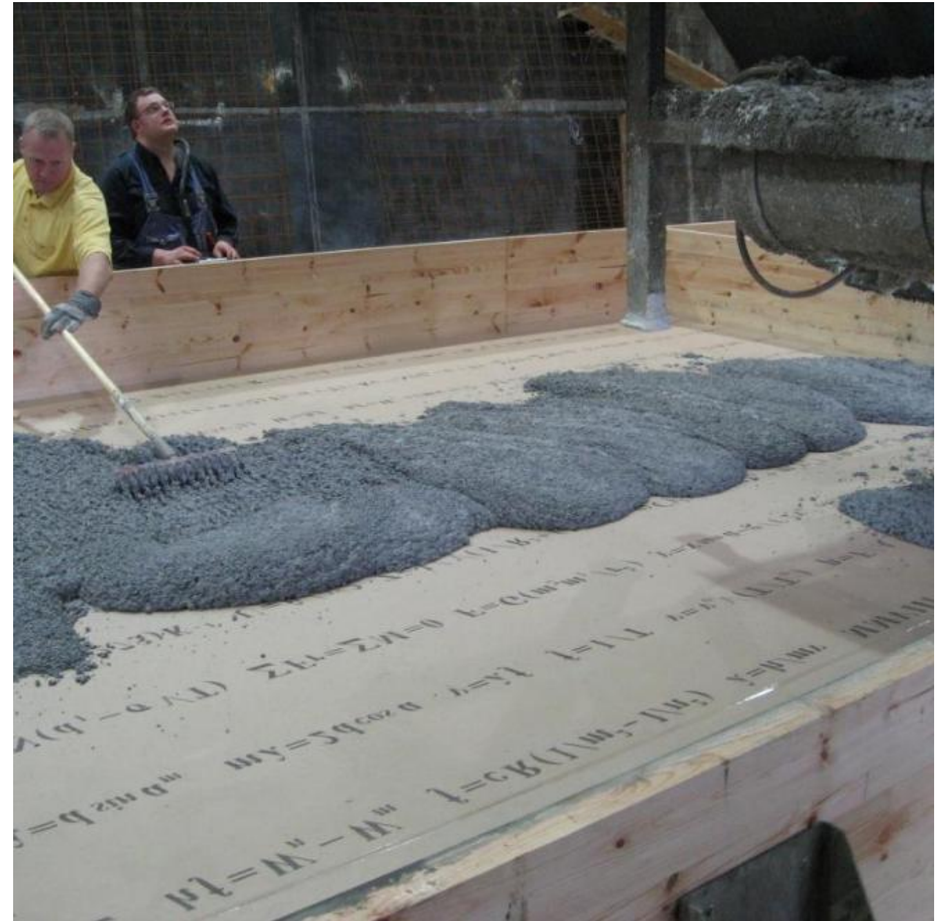
Concrete is poured (casted) on the paper.
